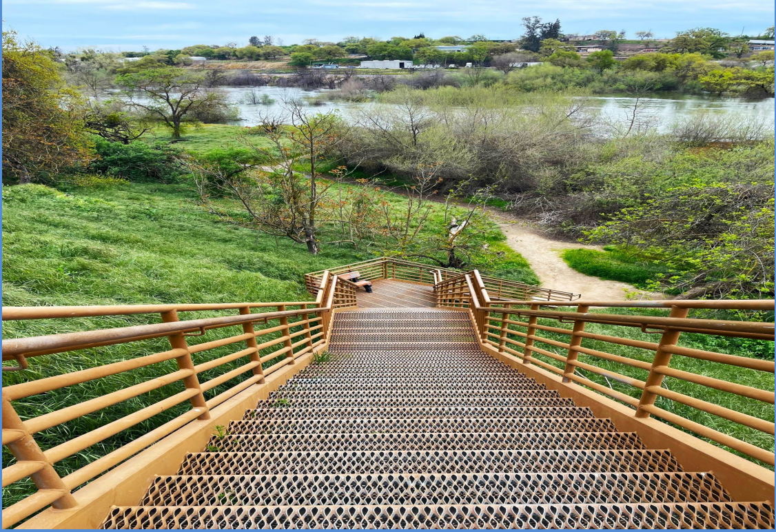
City of Waterford - Tuolumne River Staircase April 2023
