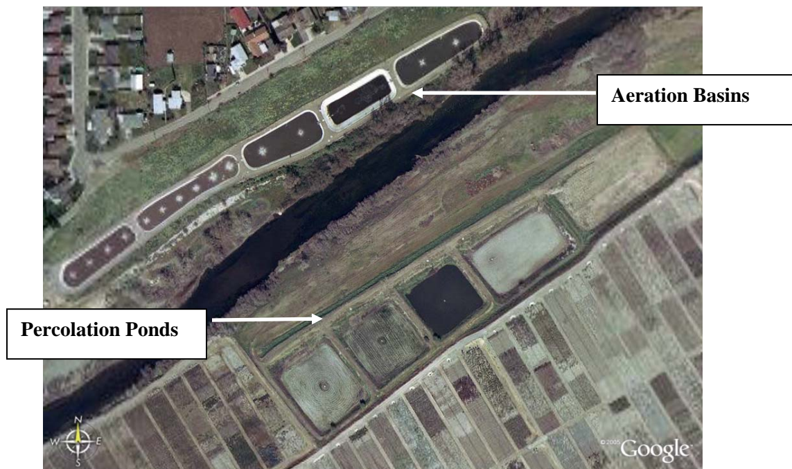
Figure 5 – Existing Waterford WWTP Site
